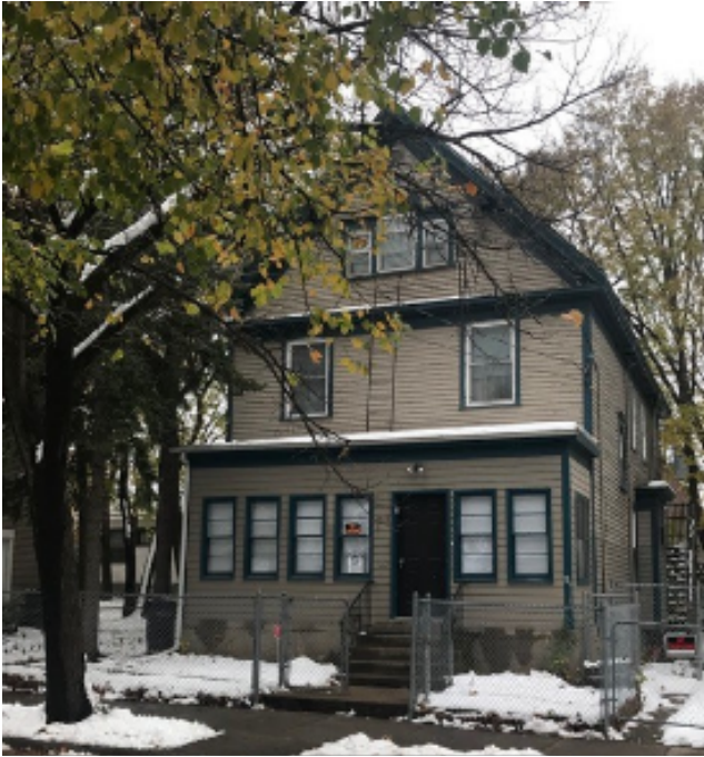
Clifton Place Apartments
